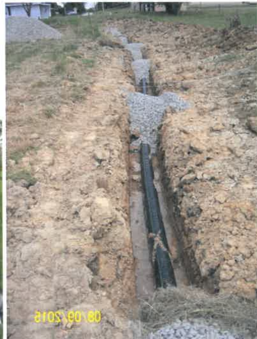
Perforated pipe surrounded in stone with straw separation layers.
