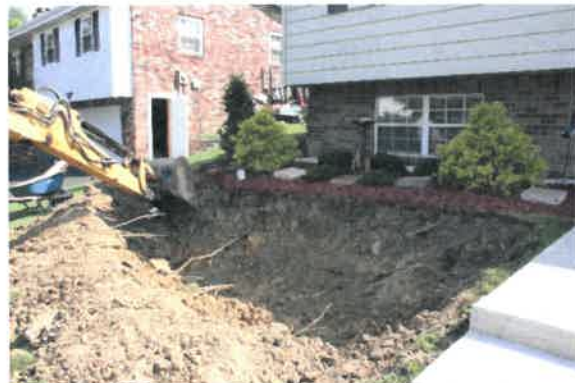
Excavate rain garden at least 10" from foundation.
