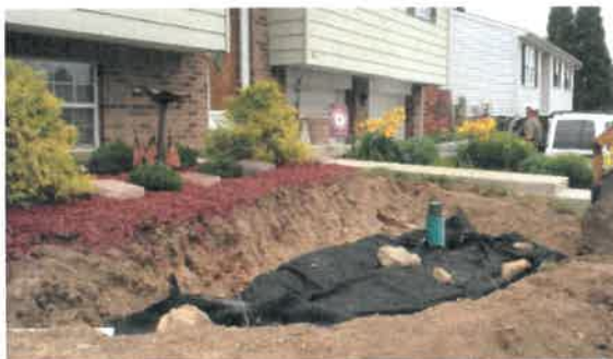
Separate bottom from soil with geotextile or straw.
