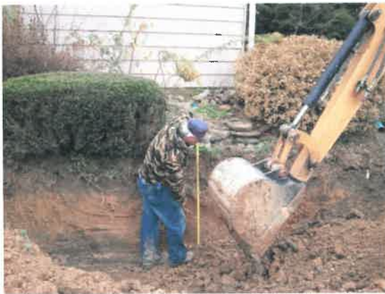
Excavate a dry well at least 10' from foundation.
