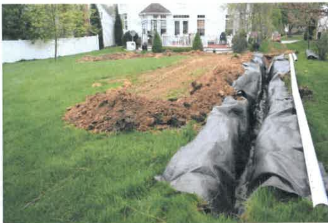
Perforated pipe surrounded with stone and wrapped in geotextile.
