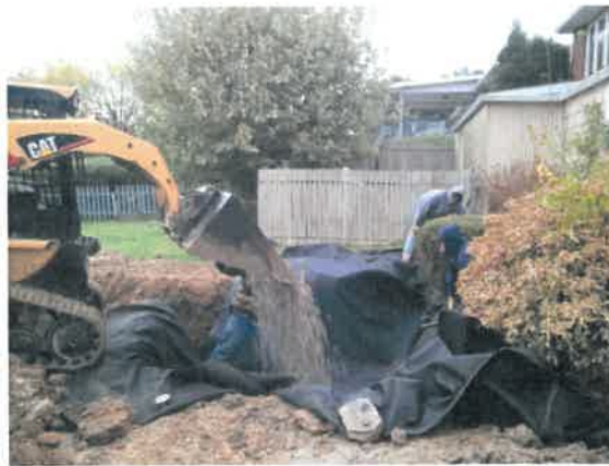
Separate stone from soil with straw layers or geotextile.
